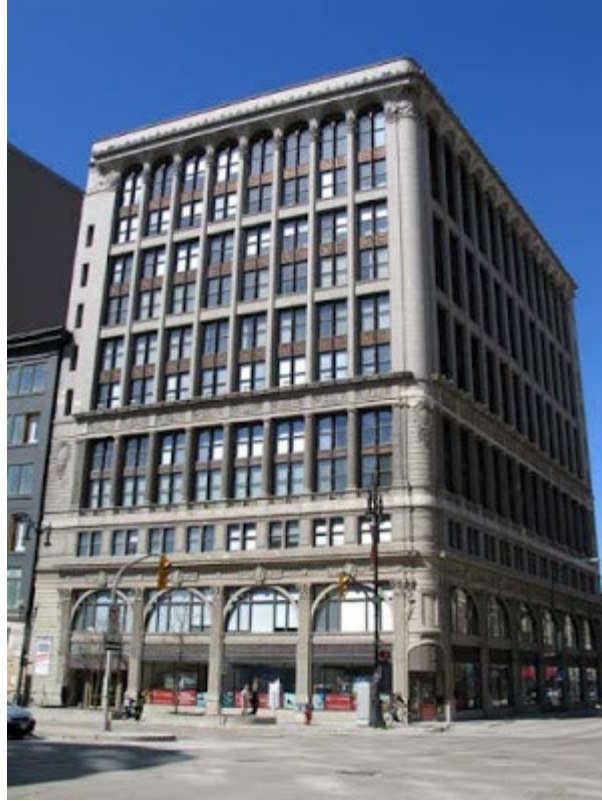
The Paris Building, present day. Built 1915 by Carter-Halls-Aldinger and designed by John Woodman and Raymond M. Carey . Source: Manitoba Historical Society
