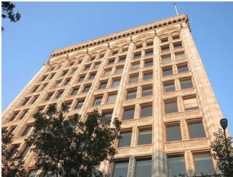
The Electric Railway Chambers Building, present day. Built 1912 by Carter-Halls-Aldinger and designed by Ralph B. Pratt and Donald A. Ross . Source: Manitoba Historical Society
